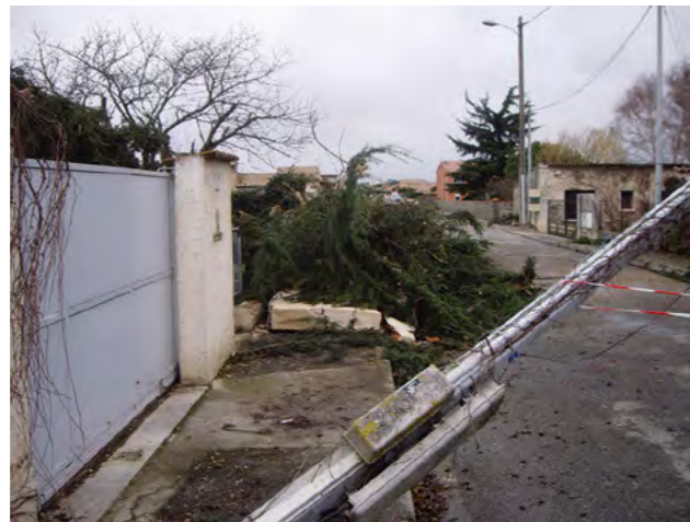
Fig. 15: Cyclone Klaus caused massive damages when it hit Southwest France in 2009, as seen here in Fonbeauzard
