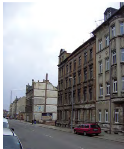
Fig. 23: A mix of brownfield, empty lots and occupied buildings on Palmstrasse in Chemnitz
